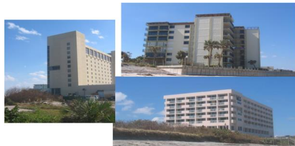
Figure 14. Examples of mid- and high-rise buildings (MHB).
