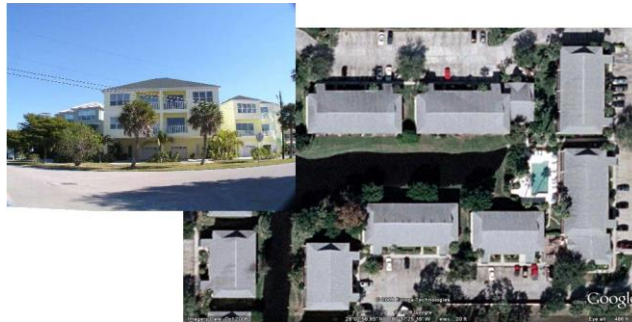
Figure 13. Typical low-rise buildings (LB).
