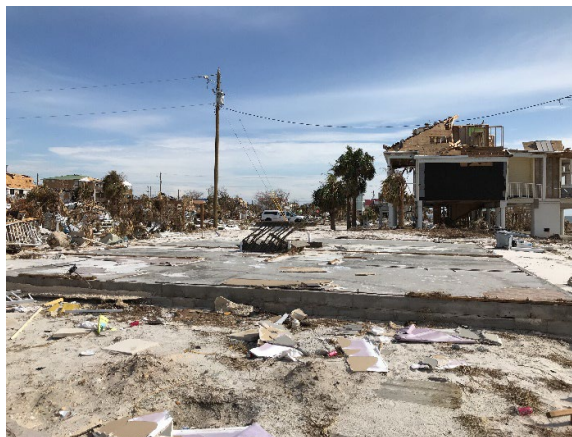
Example of residential damage after hurricane Michael, 2018
