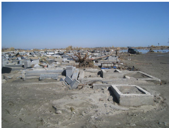
Example of residential damage after the 2011 Great East Japan tsunami
