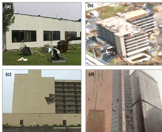
Figure 102. Damage to (a) Mechanical Equipment, (b) Roof, (c) Cladding, and (d) Windows
