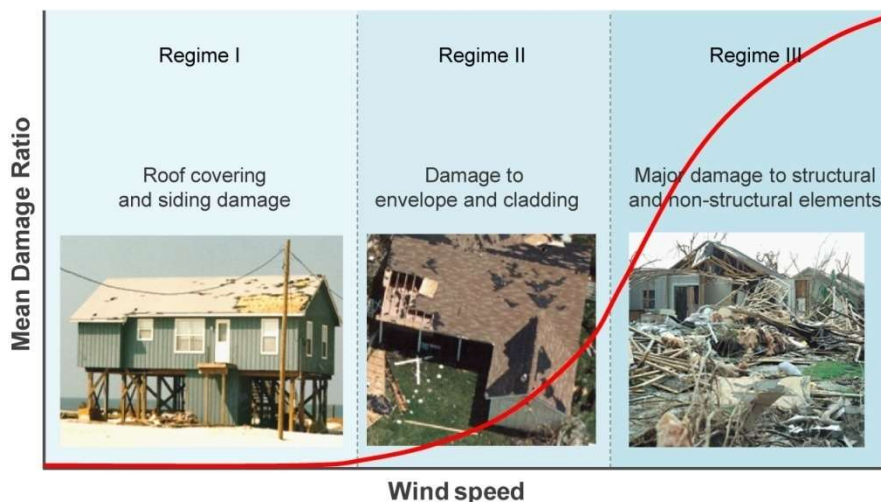
Figure 90. Damage Profile of Non-engineered Buildings
