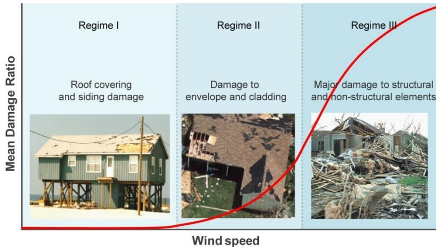
Figure 84. Damage Profile of Non-engineered Buildings
