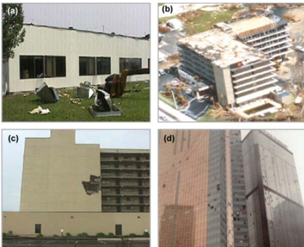
Figure 10. Damage to (a) Mechanical Equipment; (b) Roof; (c) Cladding and (d) Windows
